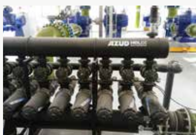
4x AZUD HELIX AUTOMATIC 4DCL9 Westbay office towers
